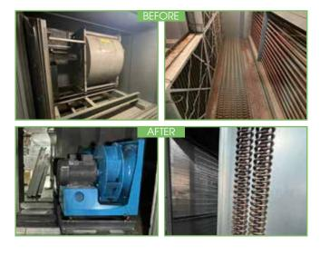
Energy Efficiency The new run around coils provides heat recovery at 68% efficiency
