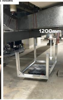
With access to the 3rd floor plantroom restricted to a 700mm doorway and under pre-installed ductwork at a height of 1200mm, a flatpack solution with separated frame with individualised panels were required for the 9m x 2.1m air handling unit. Built to achieve a minimum class L2 air leakage and incorporating run and standby supply and extract fans, the HTM O3-O1 compliant unit now provides critical ventilation to a new operating theatre at the University Hospital North Tees.
