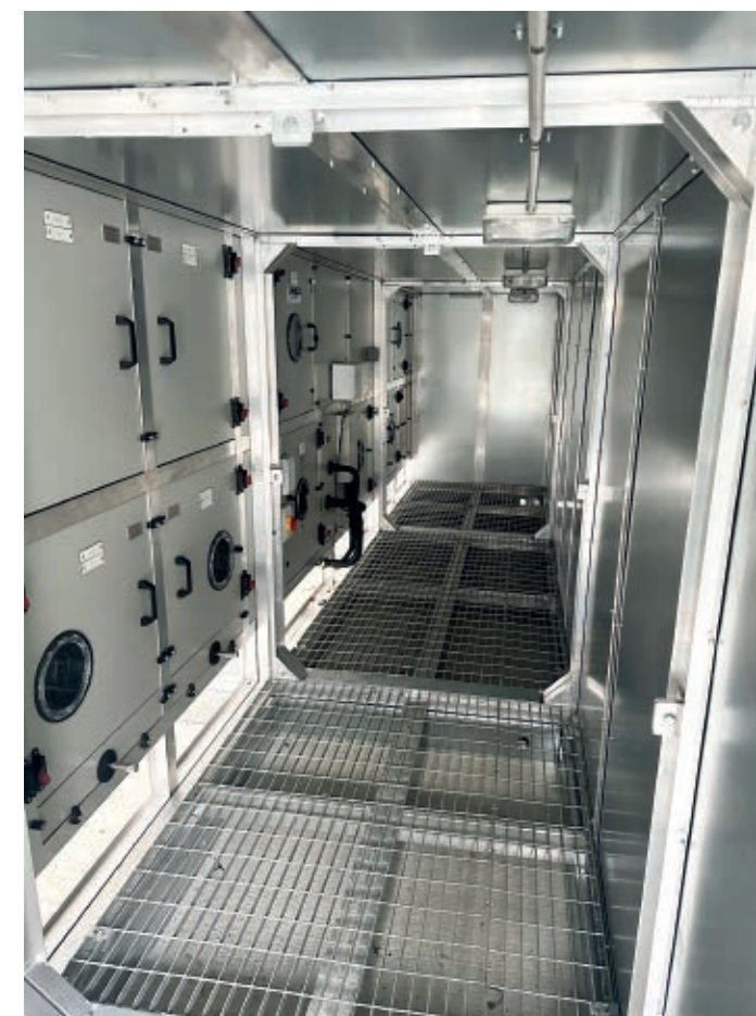
AHU with Maintenance Corridor
